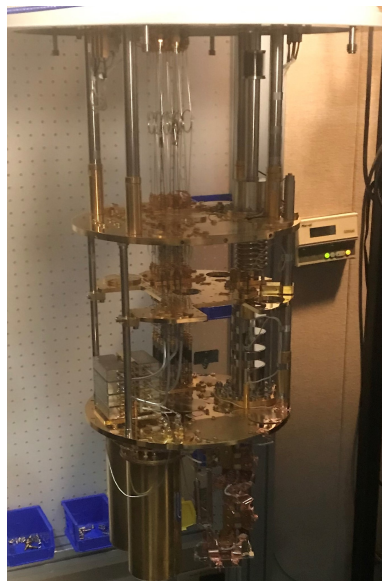
Figure 2-4: It is often useful to have an idea of the physical layout and form factor of the quantum system under testing. Each gold canister is a set of transmons inside the Bluefors dilution fridge.
